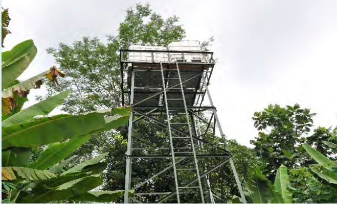
Giving support of 4 water tanks for community around Desa Kembangkuning / Bantuan 4 tanki air untuk warga Desa Kembangkuning
