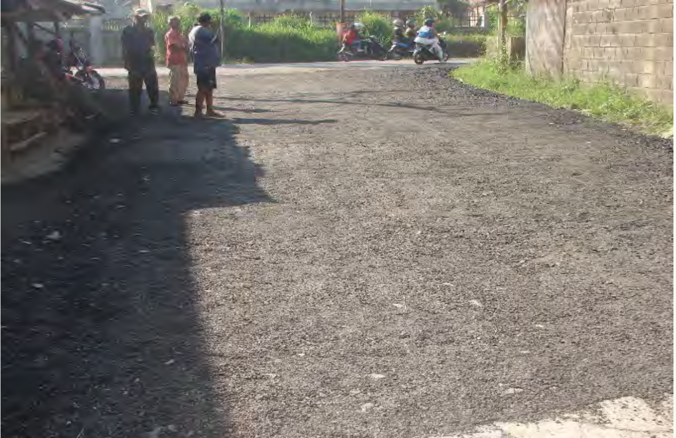
Support for Road Repairs / Bantuan Perbaiki Jalan
